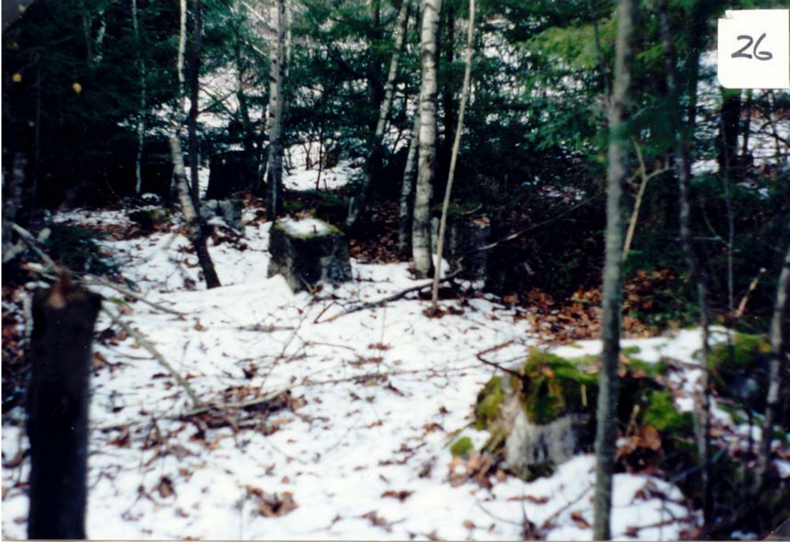
26 : This photo is looking northwest from the base of the chimney of the mill and shows some of the cement piers that supported the mill structure.
